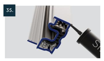
Run a continuous bead of silicone sealant around the joint between the end-milled frame and the threshold.
