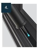
Prior to fixing the frame, silicone the holes in the bottom of the frame to prevent water ingress.
