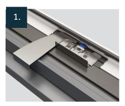
Place the de-glazing tool under the sealed unit to the back of the window section as shown. Then slide the de-glazing tool to the left / right until it meets the Securi-clip and pull towards you.
