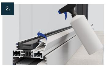
Spray the glass unit with a mild soap/water mix or glass cleaner to prevent the gasket sticking while the bead is being fitted.
