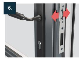
Adjust the latch plate. Backwards or forwards as shown. Then re-tighten the machine screws.
